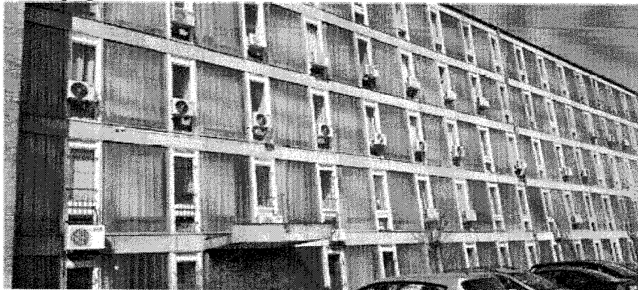
3 Fig: East façade of the Faculty of Engineering
