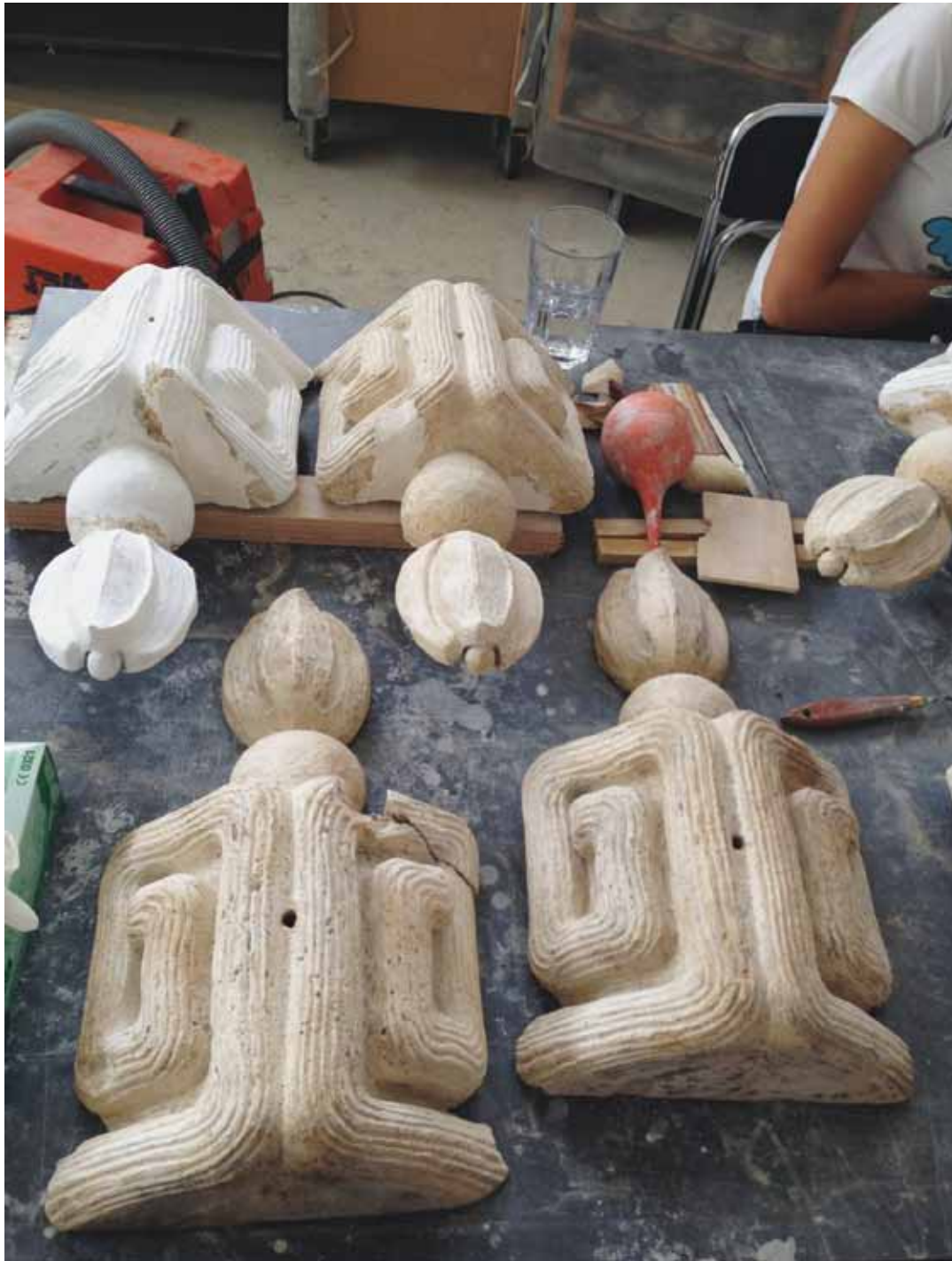
14. 80 Palmotičeva Street: Remodeled stucco elements of the entrance during the restoration
