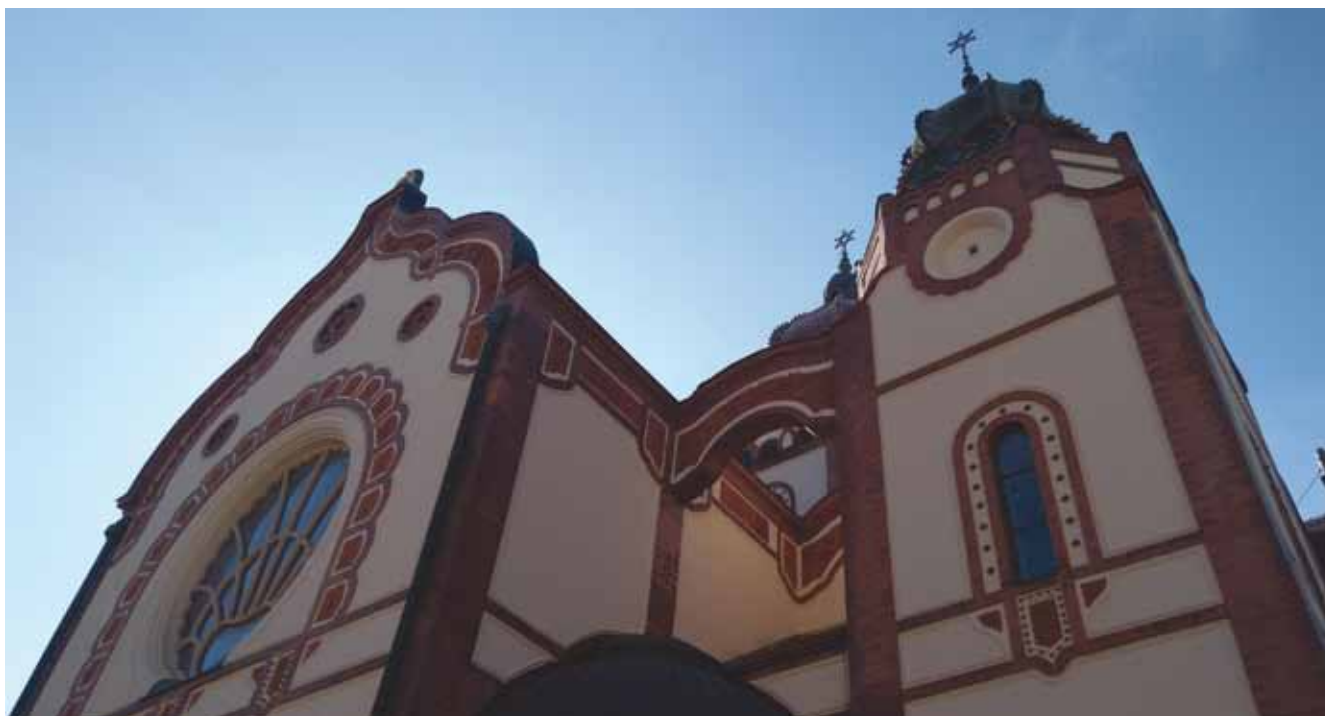
3. Northwest façade, restored in 1991
