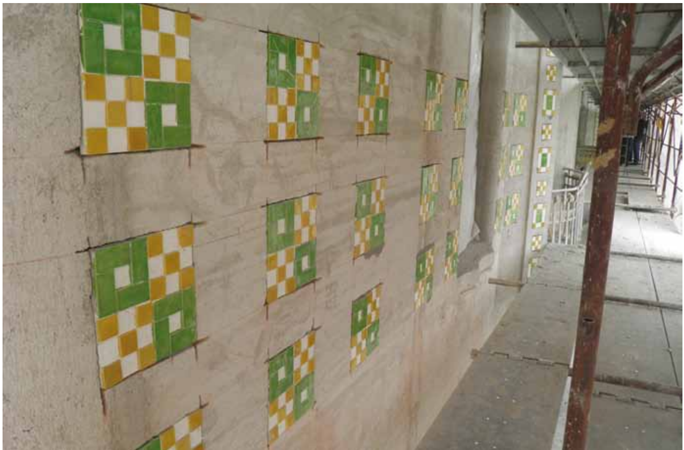
12. Adolf Moskovits Palace, the new plastering is made even with the slabs bearing the ornaments
