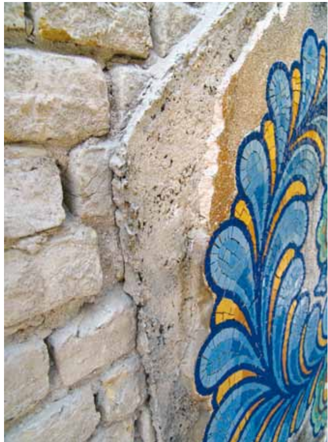
13. Layers of plaster on the primary street façade
