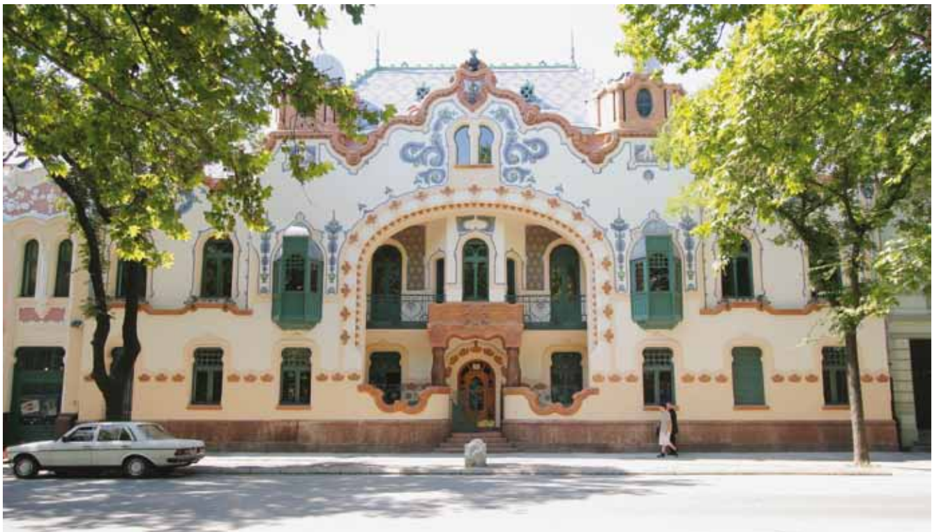
15. The primary street façade after restoration
