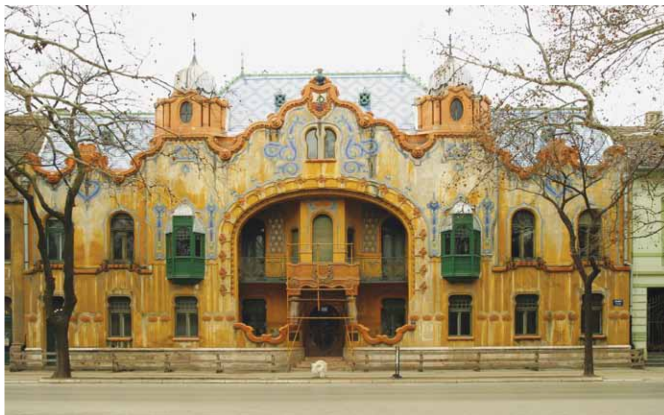
2. The primary street view of the building before the façade restoration
