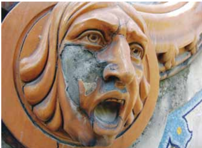
12. Damaged round human mask made of glazed ceramics from the gable of the building
