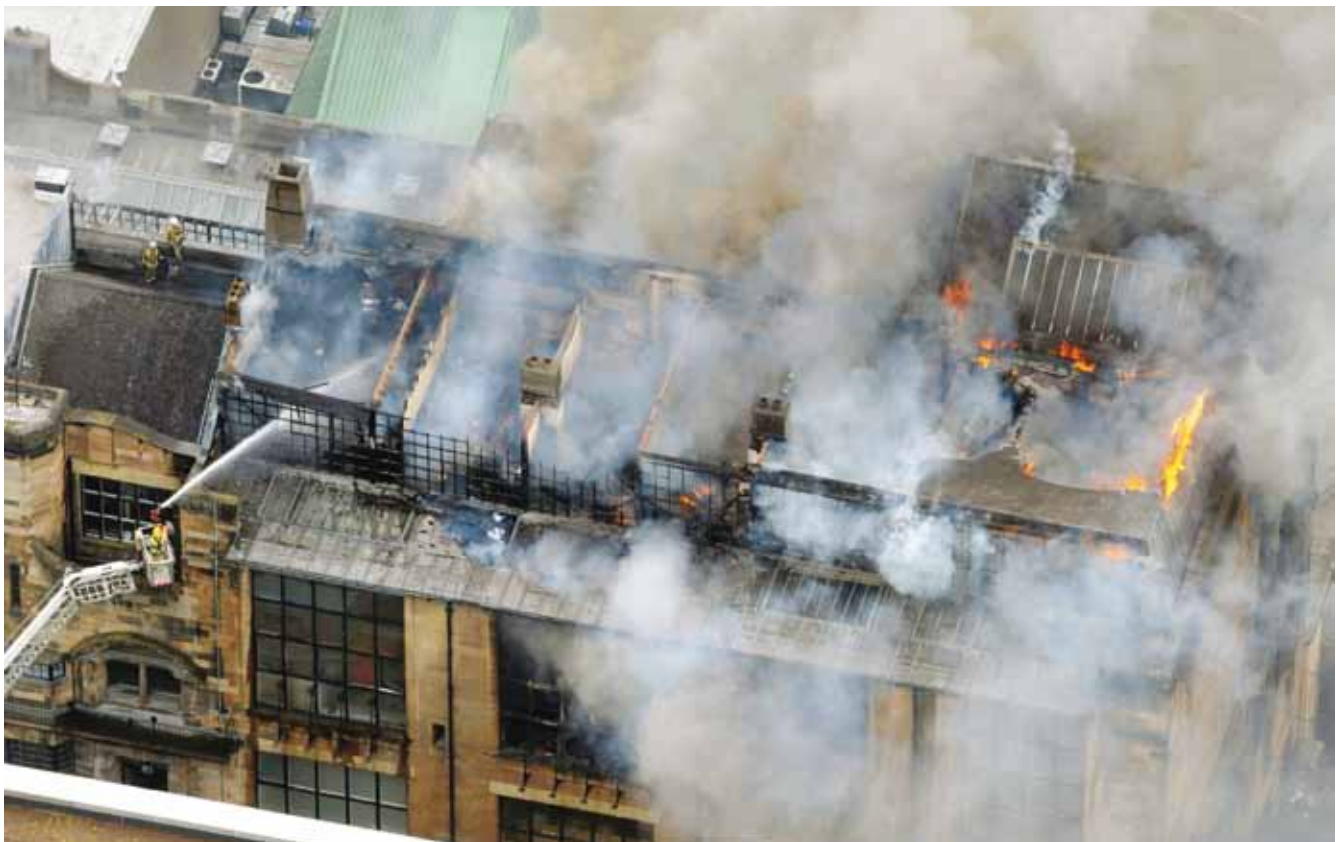
1. The fire-ravaged Mackintosh Building, 23 May 2014
