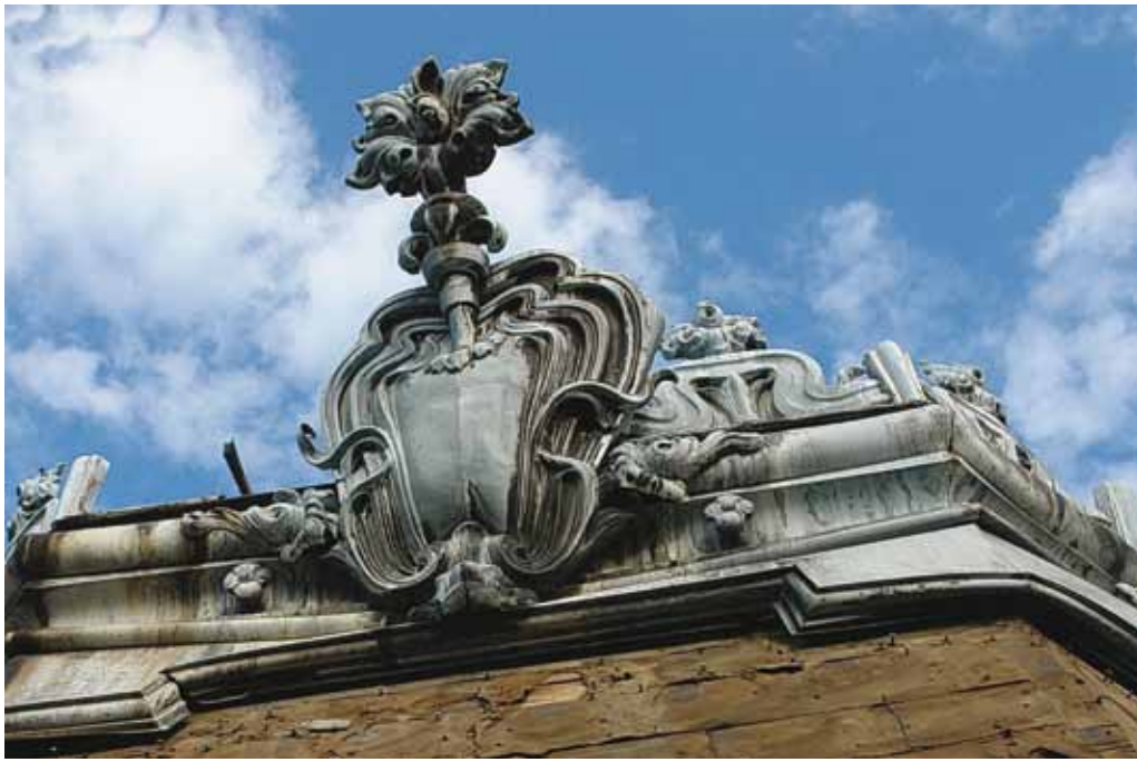
4. The Sofian House, Botoșani, Art Nouveau roof ornaments made of zinc sheets
