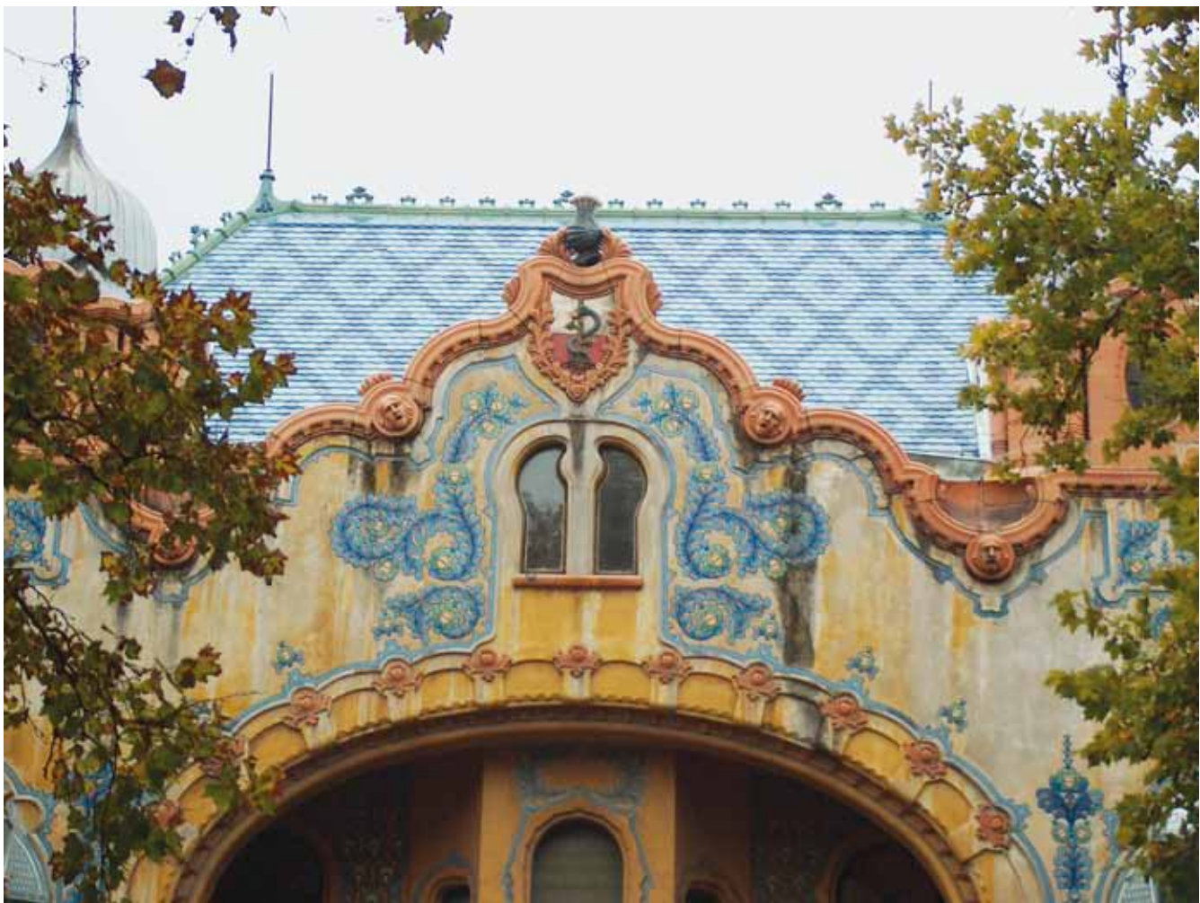
7. Detail of the roof after restoration
