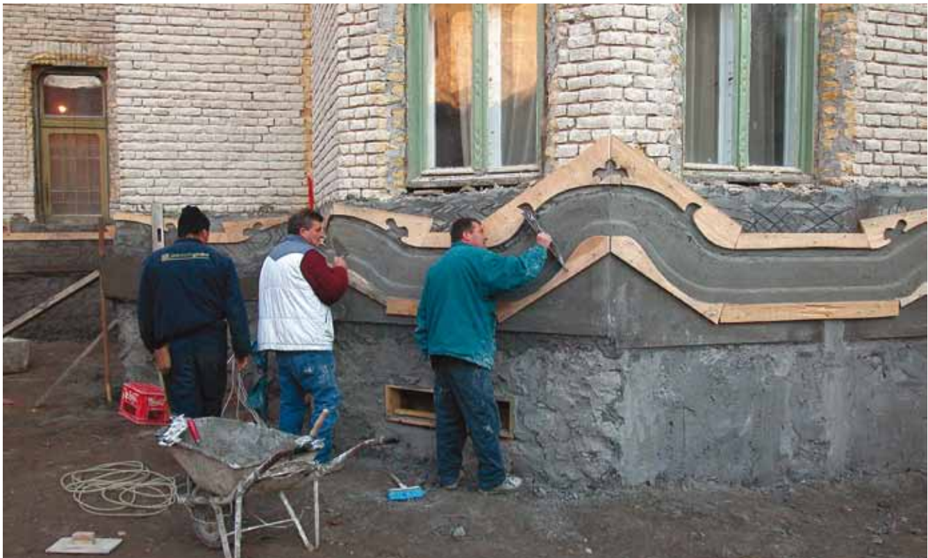
10. Restoration work on the courtyard façade using templates to make the undulating plaster forms
