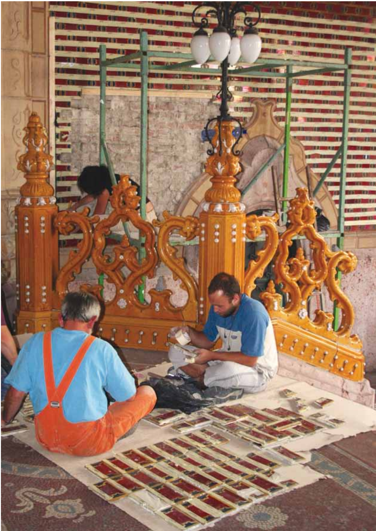
7. All the removed tiles were properly cleaned, and damaged tiles were taken to our workshop for further restoration processes
