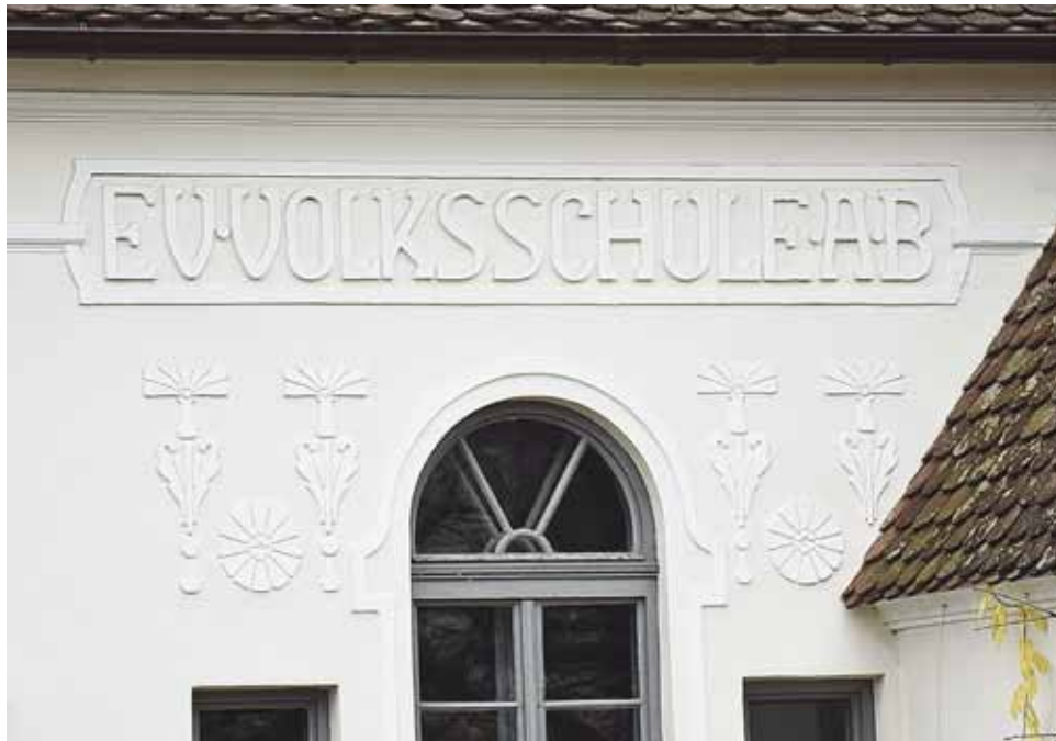
10. Former Lutheran School in Cincșor, now a conference hall, information center for rural tourism and guest house, restored Art Nouveau plaster decorations, 2017
