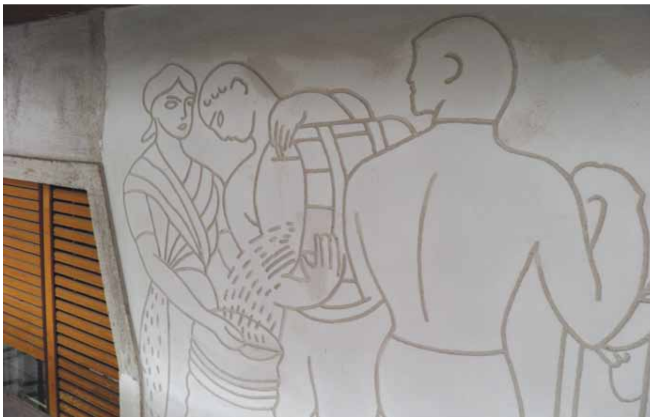
13. Adolf Moskovits Palace, sgraffito, after restoration
