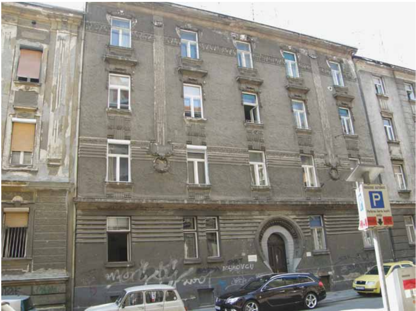
2. 20 Đorđićeva Street: Façade before the restoration
