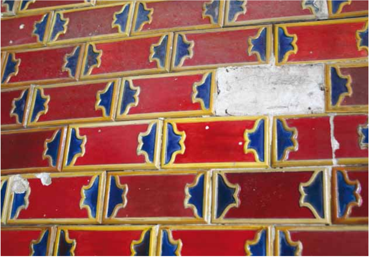
5. Decorative elements with ruby-colored luster glaze. The types of damage: gunshots, mechanical damage, damage due to leaks and fractures due to tension
