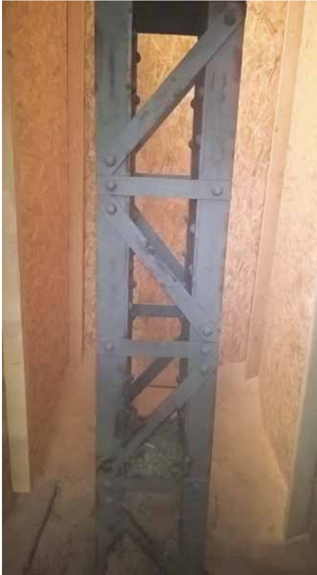
6. Cleaned iron pillar that supports the gallery and the dome, July 2017
