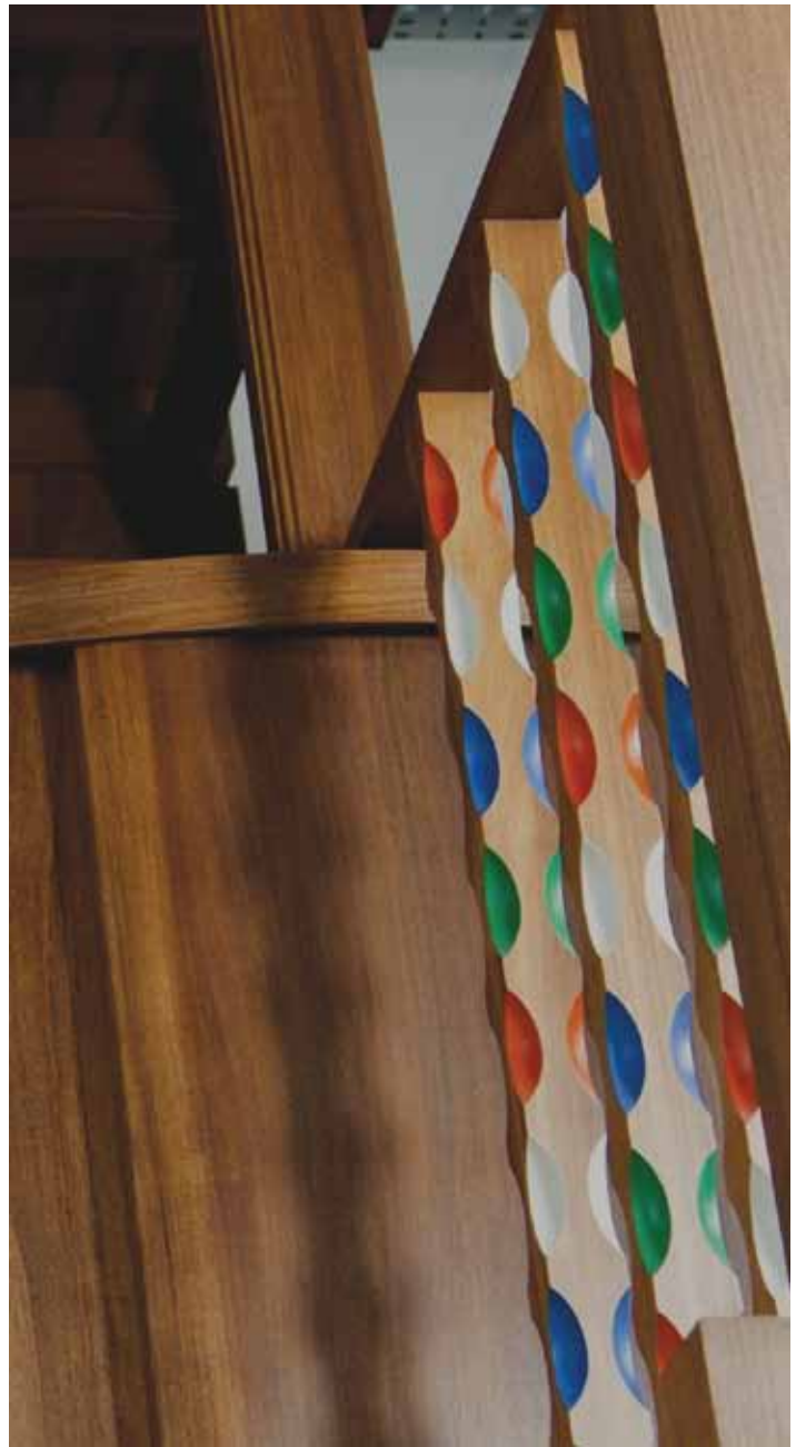
8a-b Detail of chamfered spindles, Mackintosh Library balcony (left: pre-fire c. 2012; right: Laurence McIntosh prototype model, 2017)
