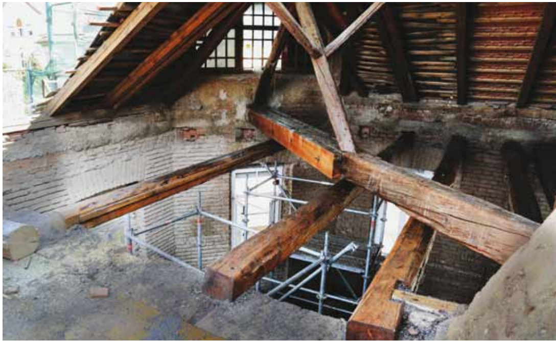
7. The edge of the roof structure
