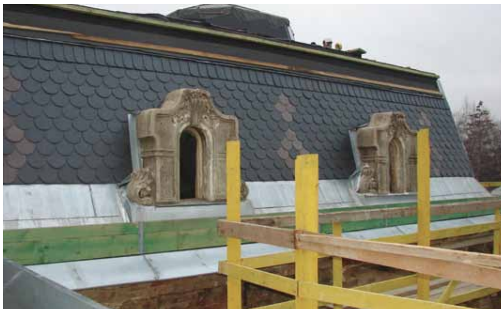
2. The Sofian House, Botoșani, roof restoration, 2016
