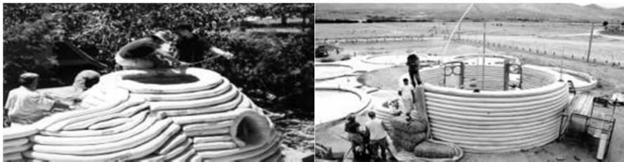
Fig. 9. The construction in the form of pots potter wrapped a method
