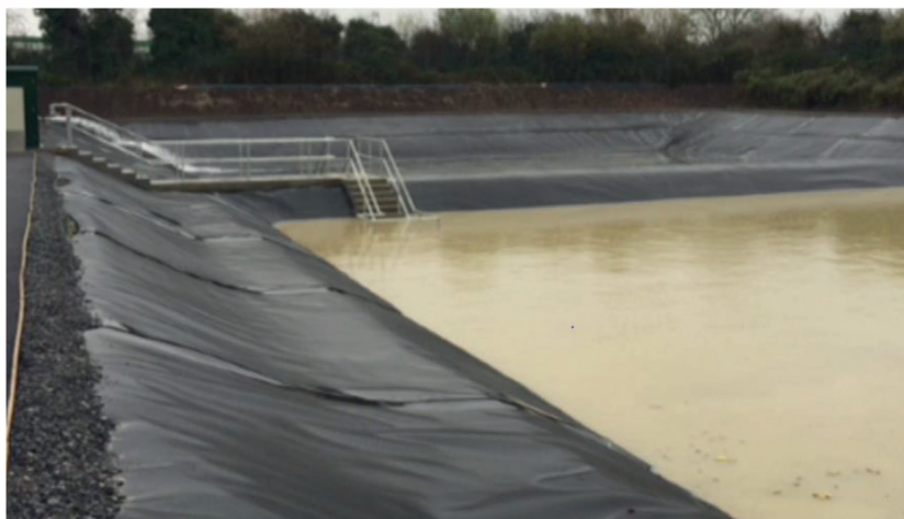
Picture 2. Fire water retention facility
