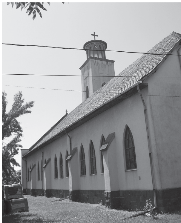
Fig. 30. Lajos Tarai (Cacinovic): Szedres, Roman Catholic church, 1948–1956, tower: 1963 (photo: Edit Lantos 2009)
