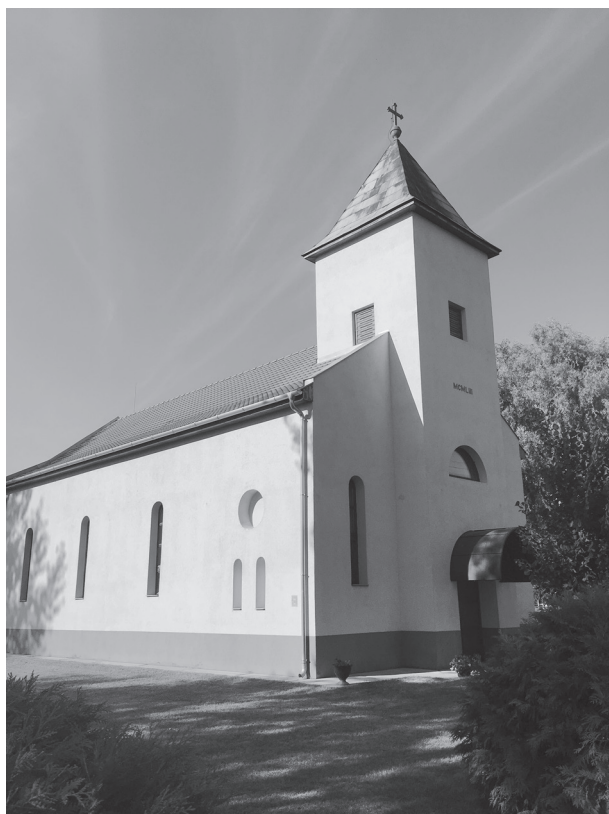
Fig. 39. Bertalan Árkay: Kömpöc, Roman Catholic church, 1949–1953 (photo: Edit Lantos 2017)
