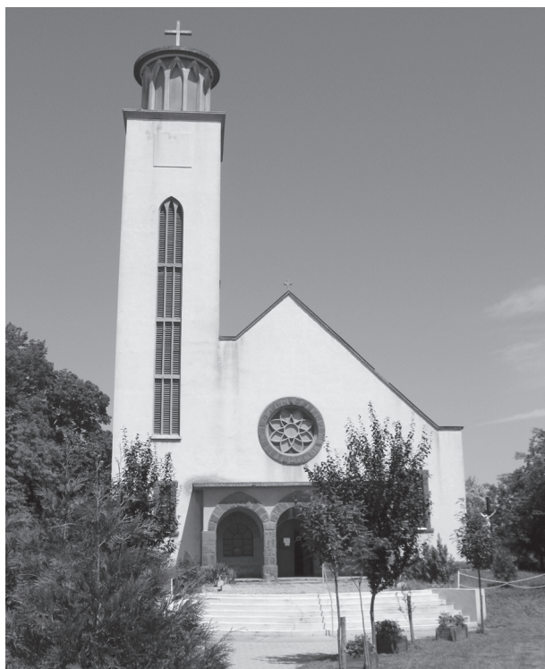
Fig. 29. Lajos Tarai (Cacinovic): Szedres, Roman Catholic church, 1948–1956, tower: 1963 (photo: Edit Lantos 2009)
