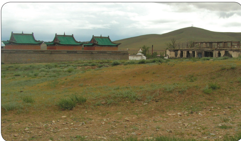
Güshig and Günreg datsan site form the North
