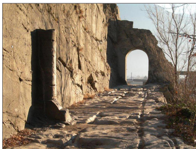
Fig. 1. Roman road cut into rock, with a milestone and a gate. Donnas, Aosta, Italy (source: http://www.crdl.scuole.vda.it/images/civilisation/paysage.pdf )
