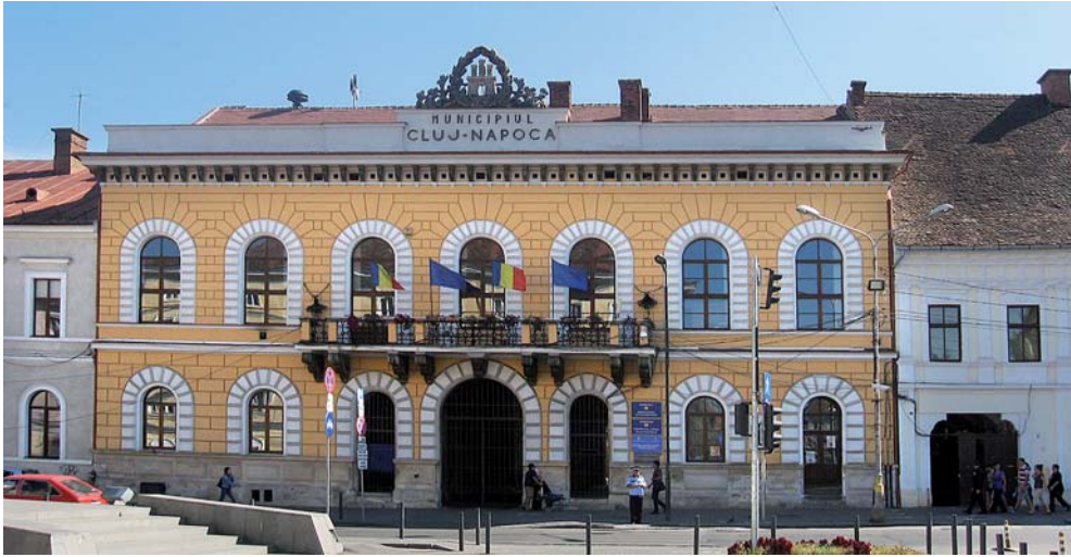
Figure 1. The old town hall built by Anton Kagerbauer between 1843–1845.
