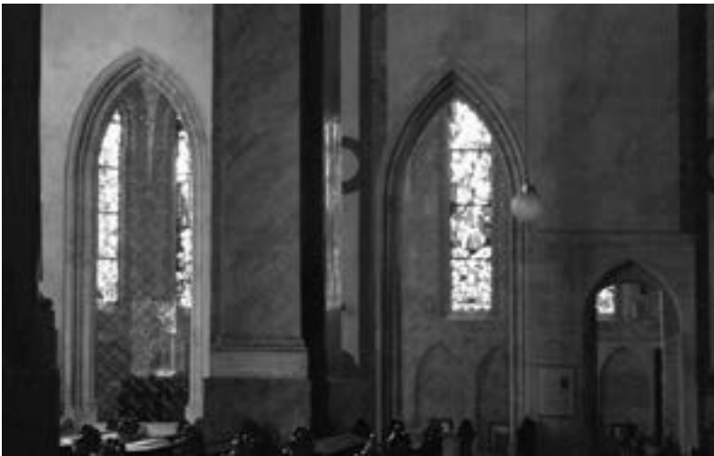
Figure 3. Győr, Holy Trinity Chapel, north wall with the two large openings
