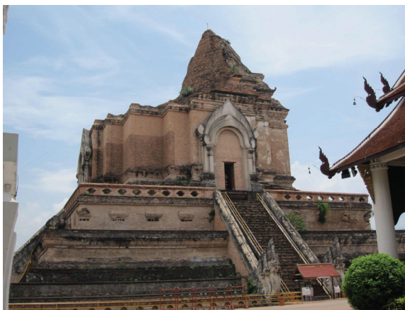
Fig. 1: Wat Chedi Luang in Chiang Mai, Thailand, seen from the southeast. Damaged during the AD 1546 earthquake, the upper half of the stupa fell to the south.
