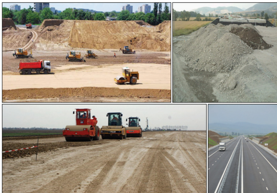
Figure 3. Using siderurgical slag aggregates for road and highway construction
