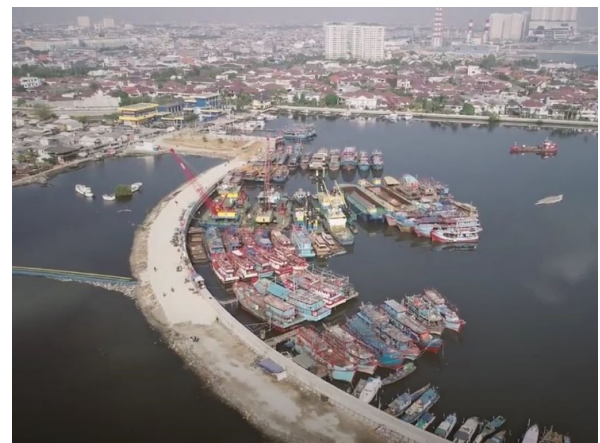
Figure 20. Inner barrier construction progress at Muara Baru.
