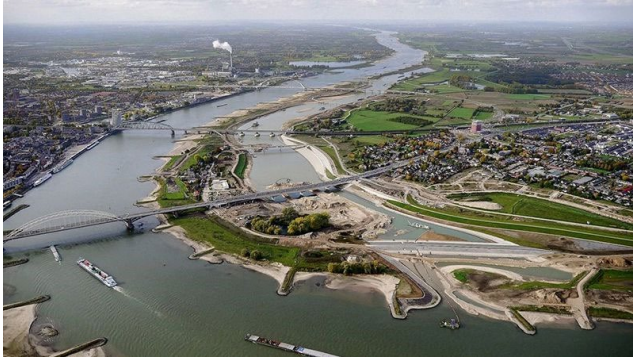
Figure 11. Room for the River, Lent, Netherlands.
