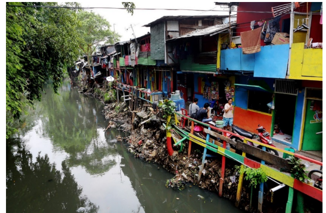
Figure 15. Typical Riverbank and Kampung at Cipinang before 'normalisation'.
