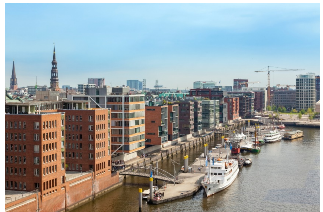
Figure 10. Sandtorhafen, HafenCity, Hamburg. Vehicle and pedestrian routes (2 levels) above flood risk height. Floating pontoons creating leisure route along the former dock.
