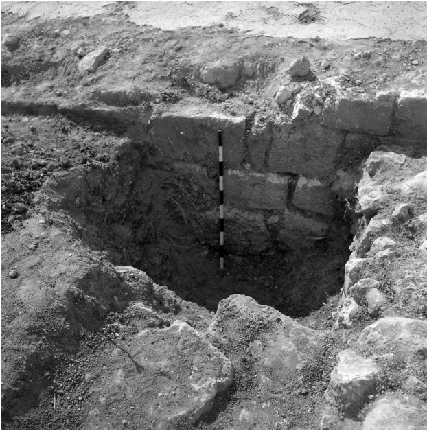
Fig. 6. Foundations walls at the western end of the northern wing (photo: Israel Antiquities Authority Photo Archive; No. 23298)
