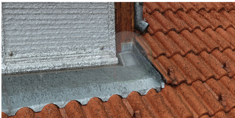
Fig. 3. Point cloud detail of the surveyed roof from images with geo-tag (Source: Olivér Rák)
