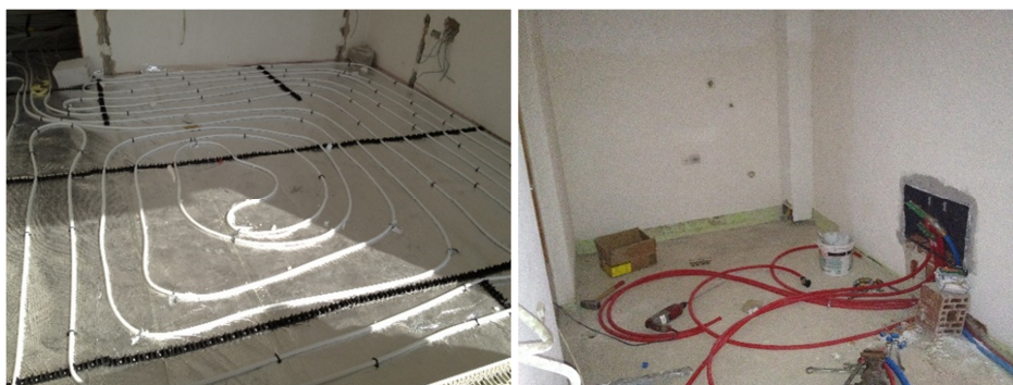
Fig. 4. Installation work (photo: Ertan Sylejmani)
