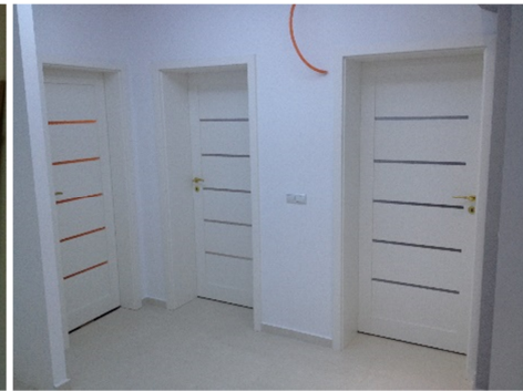
Fig. 7. Corridor after the renovation
