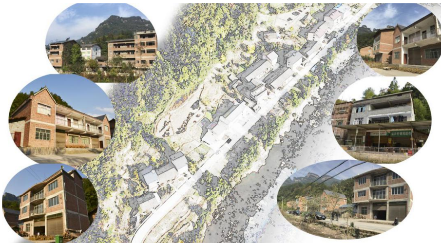
Fig. 1. Construction status of the pilot site (Source: photo and designed by Y. Shi)
