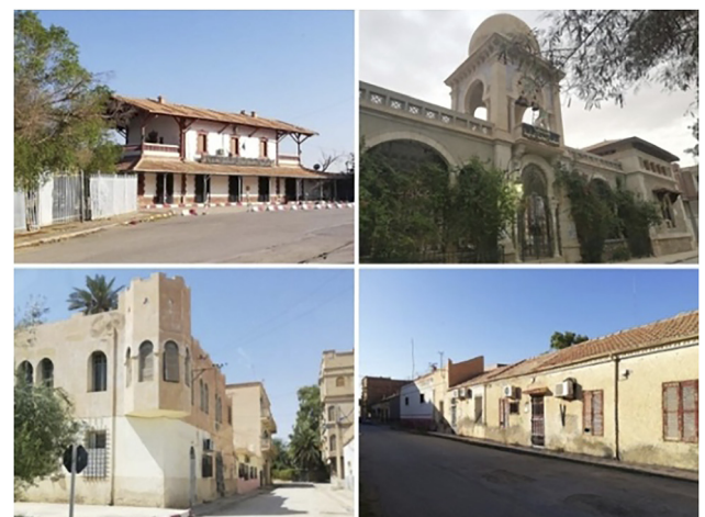
Fig. 3. Overview on some constructions in the site (Source: Author)
