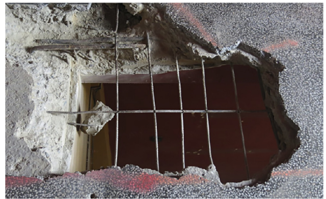
Fig. 2. Case study 1- reinforcement in the slab
