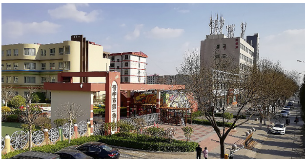
Fig. 2. Status quo of J1 kindergarten (Source: Photographed by H. Cao)
