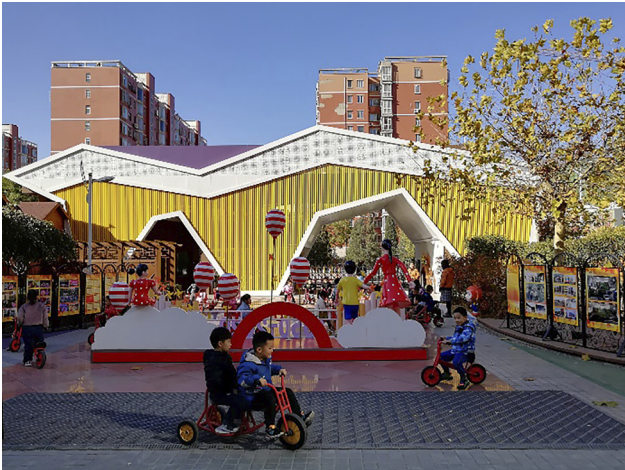
Fig. 7. The back facade of the building after completion (Source: Photographed and designed by H. Cao)
