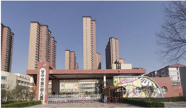
Fig. 1. Status quo of J1 kindergarten (Source: Photographed by H. Cao)
