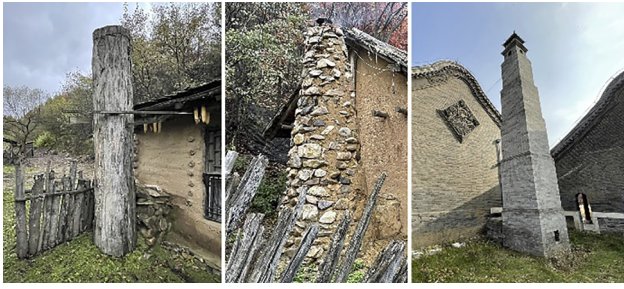
Fig. 6. Hollow tree chimney, stone earthwork chimney, stone masonry chimney (Source: photo by author)
