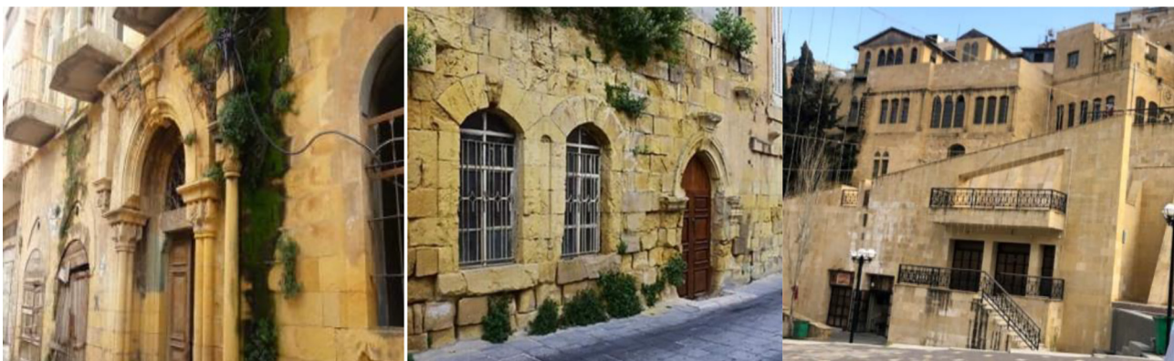
Fig. 2. Building material in Salt City golden yellow lime stone that makes the city it distinct and recognizable (Source: Author)
