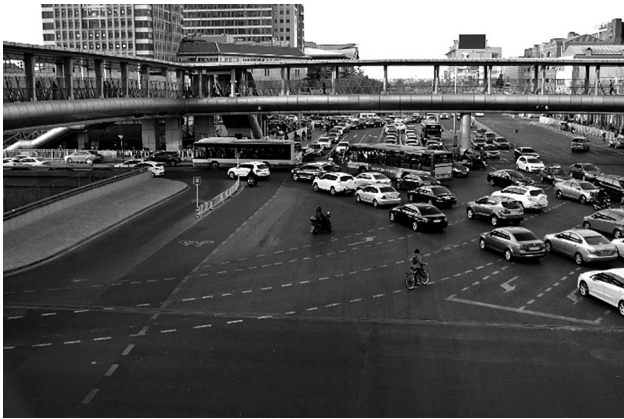
Fig. 1. Zhongguancun overpass No. 1, Beijing, China (Photo by X. Kang)
