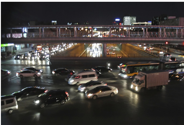
Fig. 2. Zhongguancun overpass No. 1 during off-duty hours (Photo by X. Kang)
