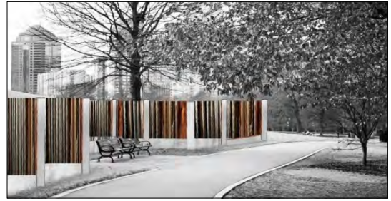
Figure 1. Three-dimensional model of noise-shielding wall: base material: wood, porcelain, ceramic, glass [2]
