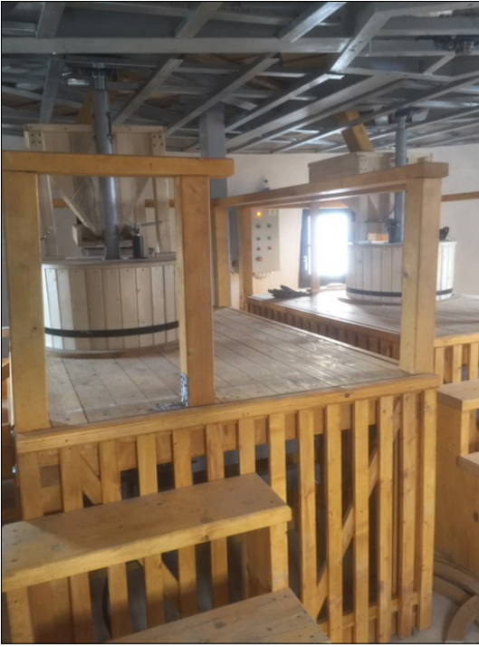
Figure 13. The machinery on the first floor.
