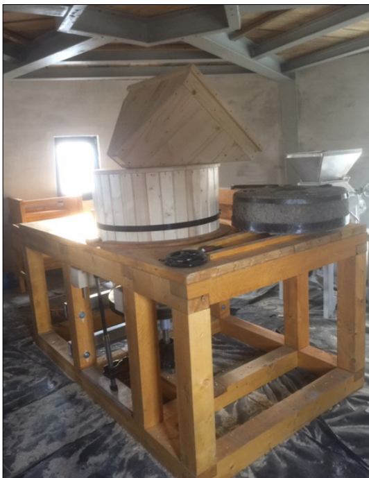
Figure 7. The windmill during installation.
