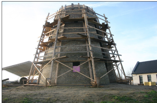
Figure 5. View of the Felsőszentiván windmill under reconstruction.
