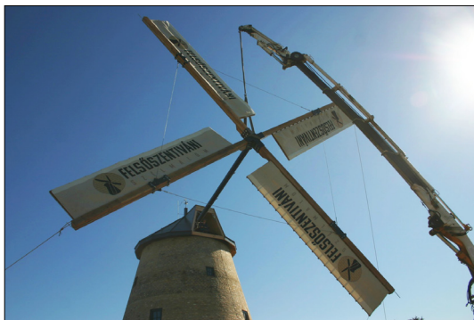
Figure 6. Lifting and repairing the wind wheel.
