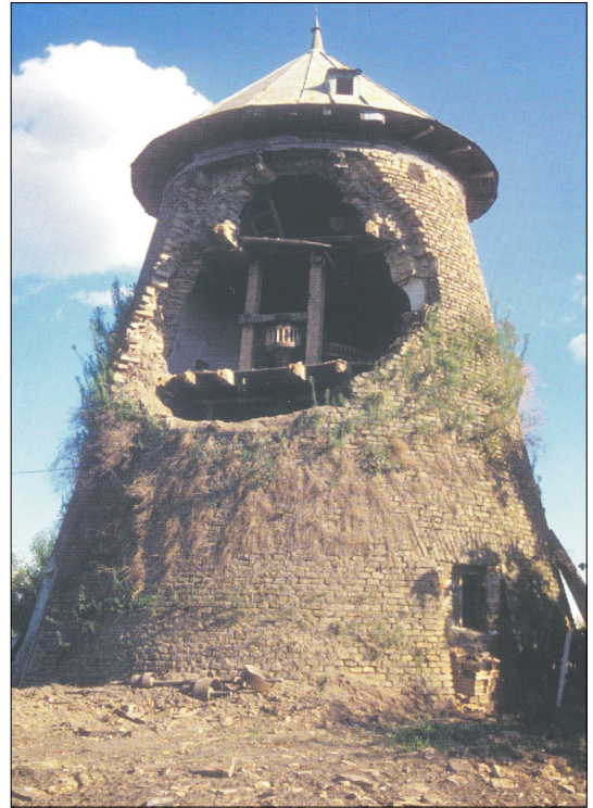
Figure 3. View of the Felsőszentiván windmill before reconstruction.
