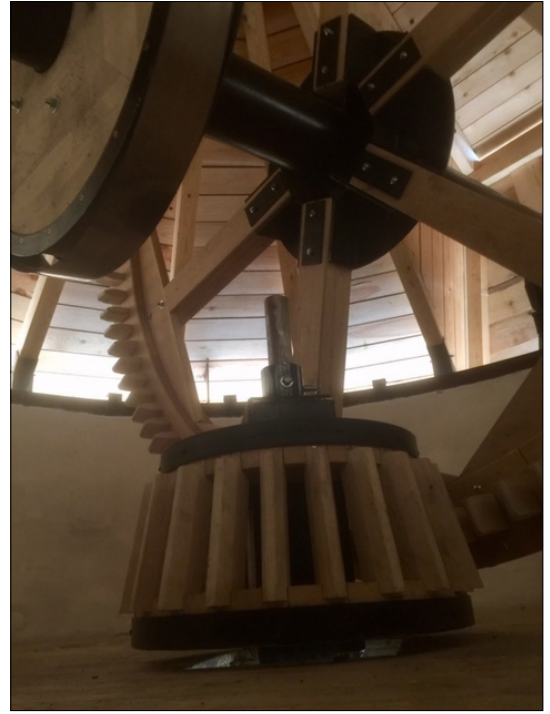
Figure 15. The machinery of the fourth floor.
