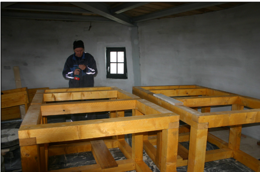
Figure 10. Assembly of the support structure of the mill machine.
