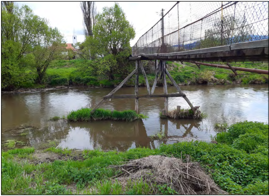
Figure 3. Pedestrian bridge on the original substructure
