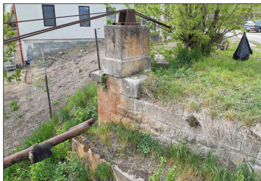
Figure 2. Ahe current state of the abutment
