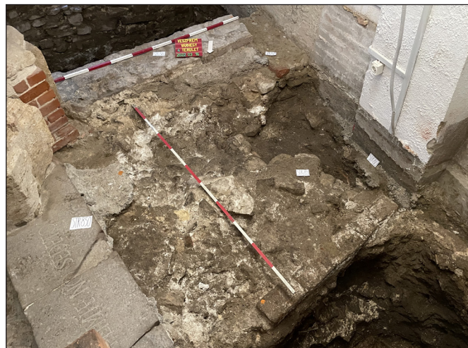
Fig. 5. Core of a dismantled wall at the entrance of the octagonal chapel
