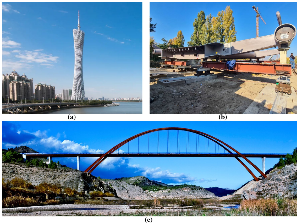
Fig. 1 Application of CFST elements in a high-rise buildings (Canton Tower, 2022) and b footbridges and c road bridges (La Vicaria bridge 2022)
