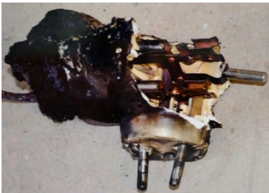
Figure 1. Galvanic corrosion affected damage
