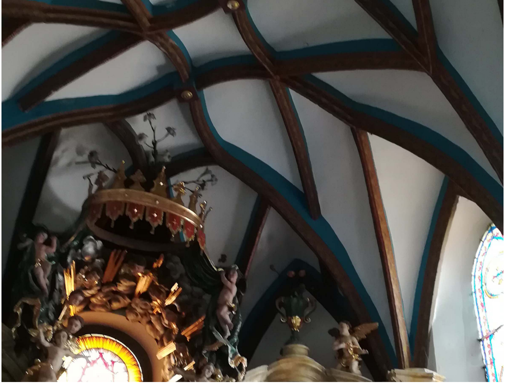
Figure 22. The connection of the E1.3 element (big profile) and the C1.6–G1.0 elements (small profile) in photo
