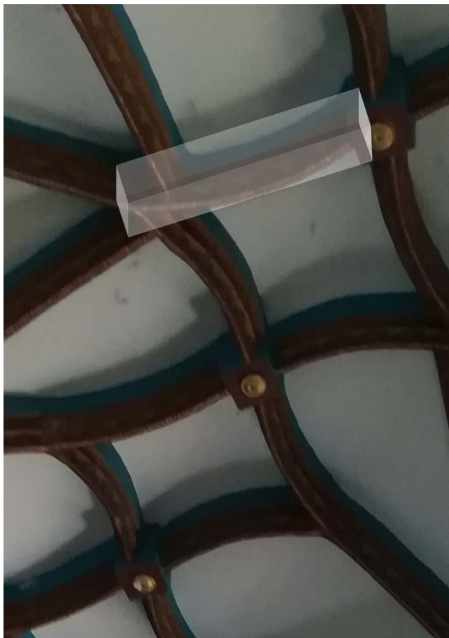
Figure 24. The theoretic overall dimensions of a curvilinear rib, represented in the photo of the vault. (Naturally, the carving of the ribs happened before they were built in, the figure only means to picture the supposed dimensions.)
