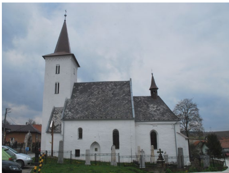
10. Spišský Hrušov/ Szepeskörtvélyes, parish church, south façade (photo author, 2017)
