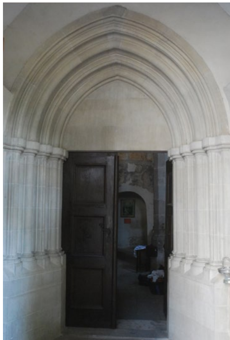
9. Poprad/Poprád, parish church, the reconstruction of the south portal (photo author, 2015)
