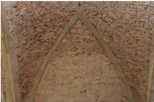
4. The chancel's second wall-shaft from the West with the trace of the 18th century vault and the reconstructed pointed arch and caps, 2020. Photo by Radu Lupescu.
