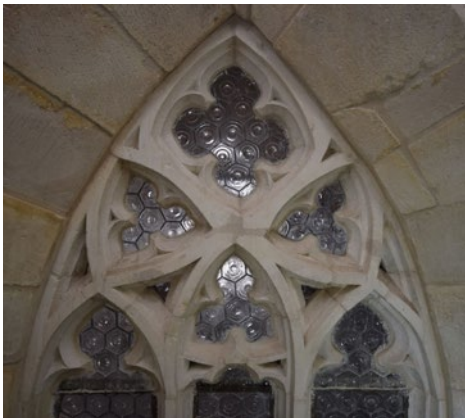
8. The reconstructed tracery on the south side, 2021. Photo by the author.
