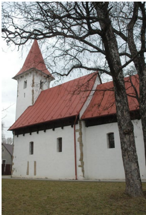
8. Mengusovce/Menguszfalva, parish church, the restored church from south-east (photo author, 2014)
