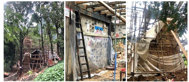
Fig. 7. Protection of trees and old wall in construction (Source: photo by Shi Yongting)
