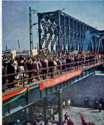
THE MAIN RAILWAY BRIDGE over the Danube at Budapest is opened, and workers who helped in its rebuilding walk across behind the first train. Banner on bridge reads: "Long Live the Soviet Union, Strongest Guardian of Peace."
