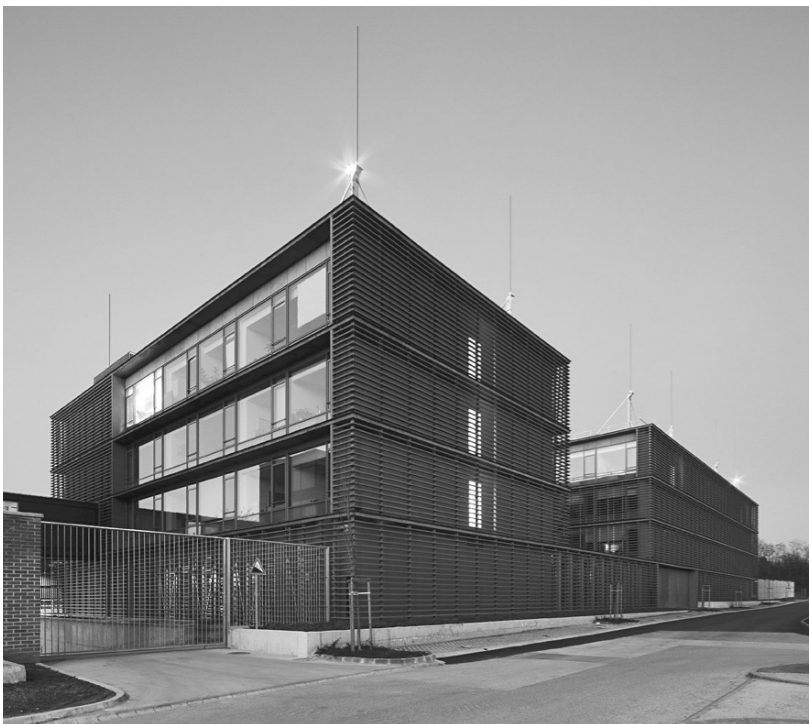
Photo Foto: Tamás Bujnovszky http://ad009cdnb.archdaily.net/wp-content/uploads/2013/04/5153bc2cb-3fc4b4783000049_center-of-air-navigation-services-zsk-architects-_hc-_234.jpg
