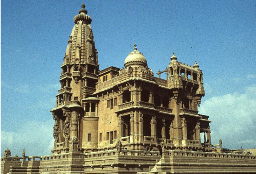
Fig. 10. The Palace of Baron Empain, general view.
