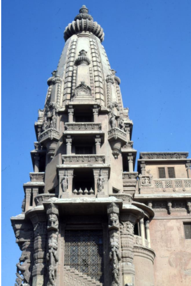
Fig. 11. The Palace of Baron Empain, tower.
