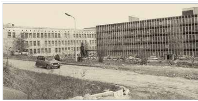
Area pertaining to today's building A/6, with building A/4 in the background. (Source: The archives of Prof. Dr. Miklós Szabó)
