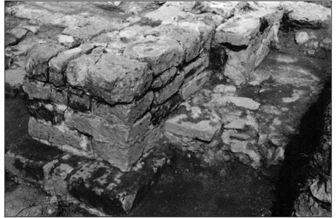
Fig. 7. The ashlar masonry of the double arched gate of the large western tower in 1971 (Photo by Mátyás Szőke and Sándor Soproni)
