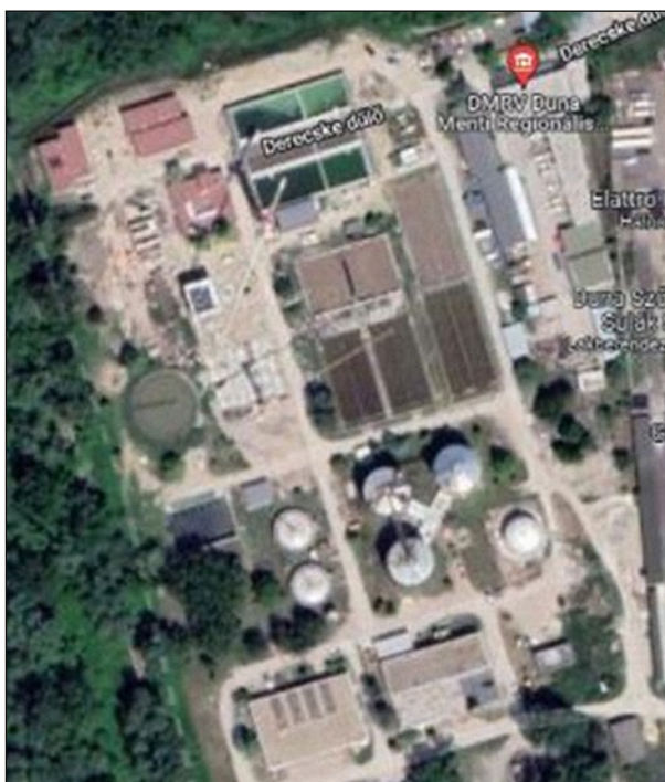
Picture 5: Top-view of the WWTP
