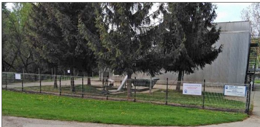
Picture 8: One element of the fence on the northern section of the WWTP
