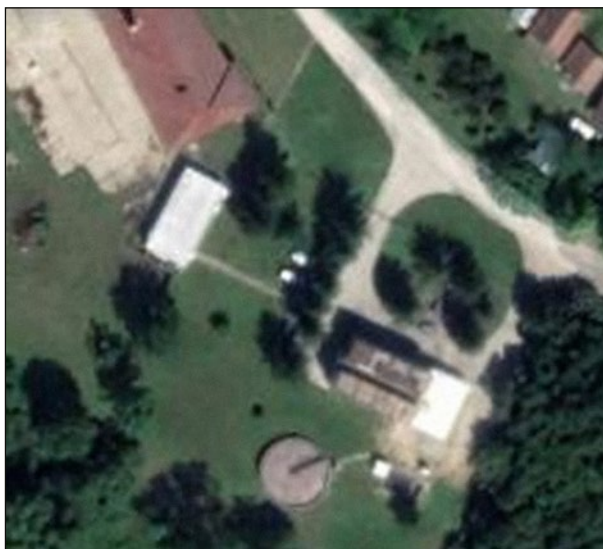
Picture 7: Top-view of the WWTP
