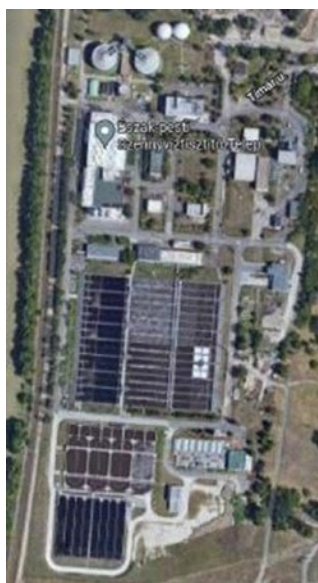
Picture 1: Top-view of the sewage treatment plant
