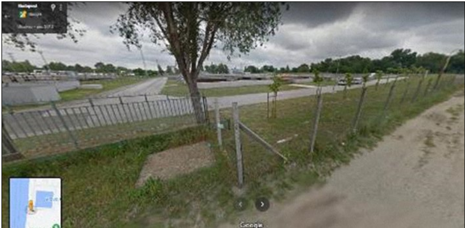
Picture 2: Fence section on the west side of the sewage treatment plant
