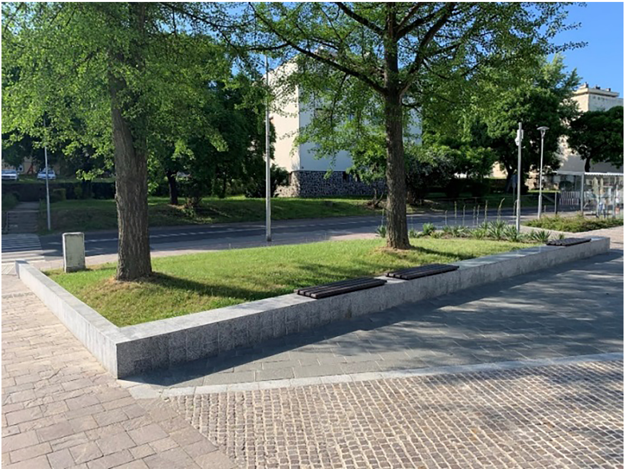
Fig. 5. Green island, granite and porphyry paving and benches of the square (Source: authors' photo)
