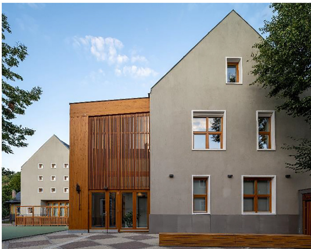
Fig. 4. Window allocation of the gable walls on the western façade (Source: photo by György Palkó)
