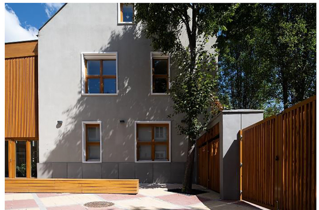
Fig. 9. The new timber-concrete main gate and the fine concrete plinth of the school (Source: photo by György Palkó)
