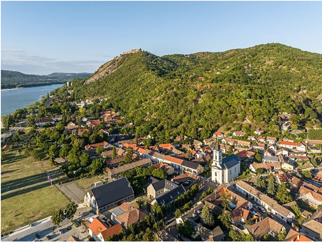
Fig. 1. Aerial view of the downtown of Visegrád with the primary school and the citadel in the background (Source: photo by György Palkó)
