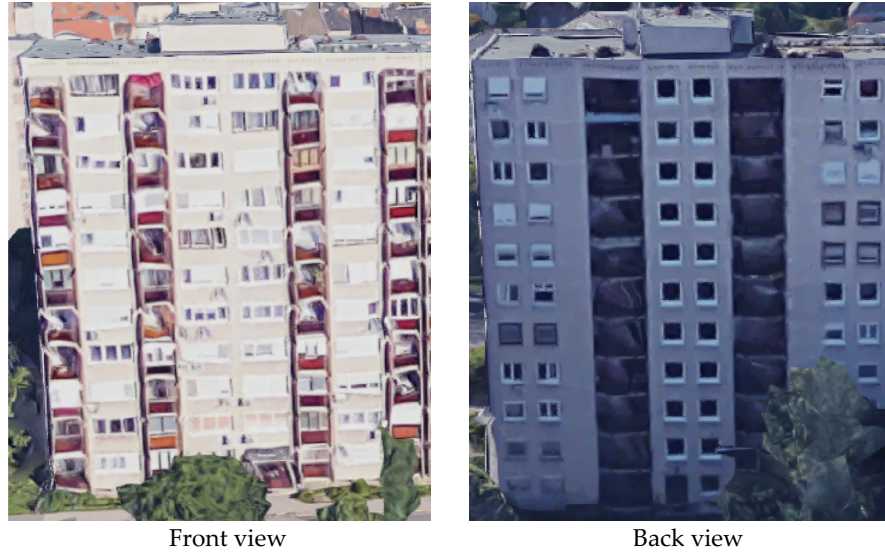
Fig. 1. Type 1 building front and back view.
