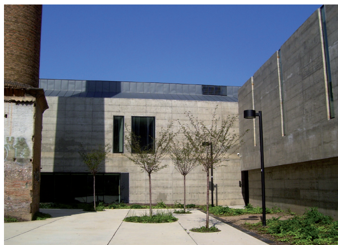
Fig. 4. Can Framis Museum, Barcelona 2008. Architect: BAAS Arquitectos. Picture: author
