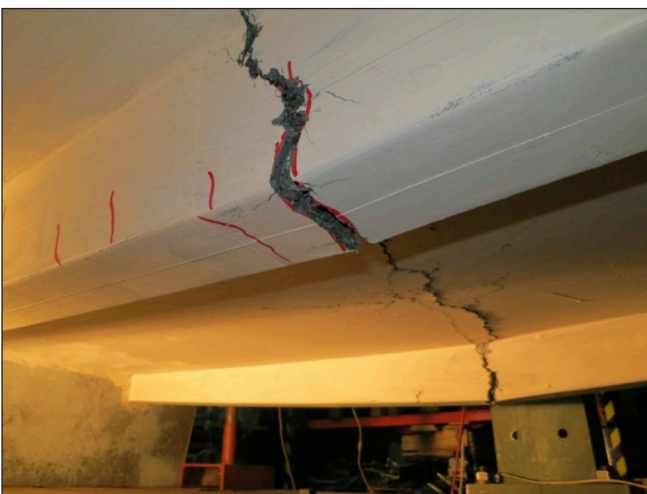
Fig. 7: Failure of the model in transversal bending
