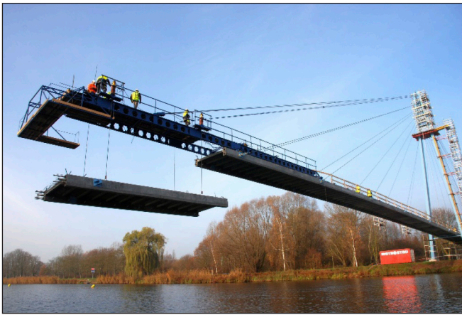
Fig. 14: Assembly of the segments in the main span
