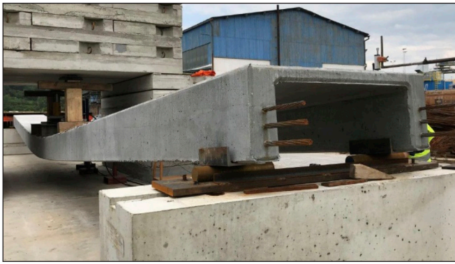
Fig. 11: Loading test of a pretensioned beam
