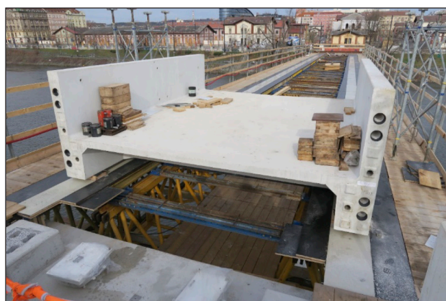
Fig. 24: Typical segment of the footbridge in Prague (2023)
