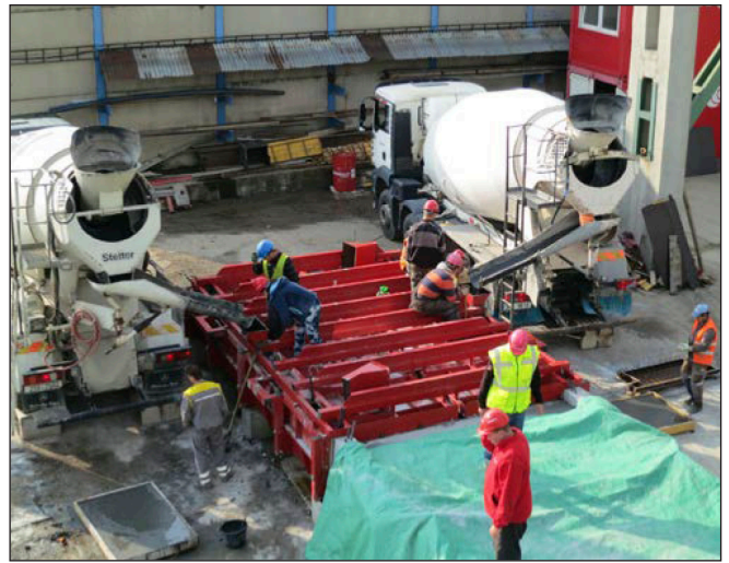
Fig. 13: Filling of the mould by UHPC from 2 truckmixers
