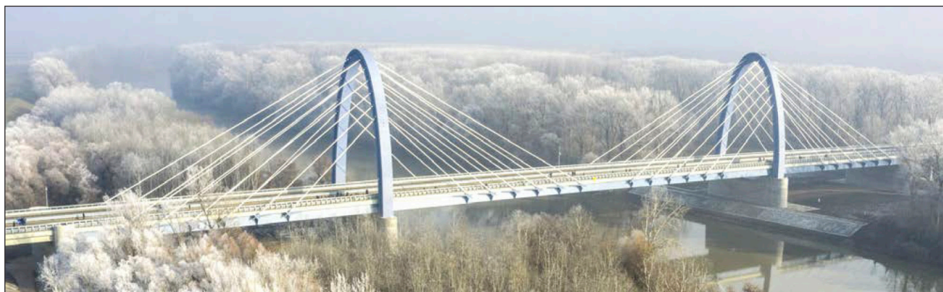
Fig. 8: The bridge from the air after its opening
