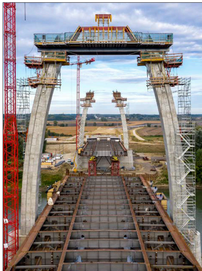
Fig. 4: Pylon under construction
