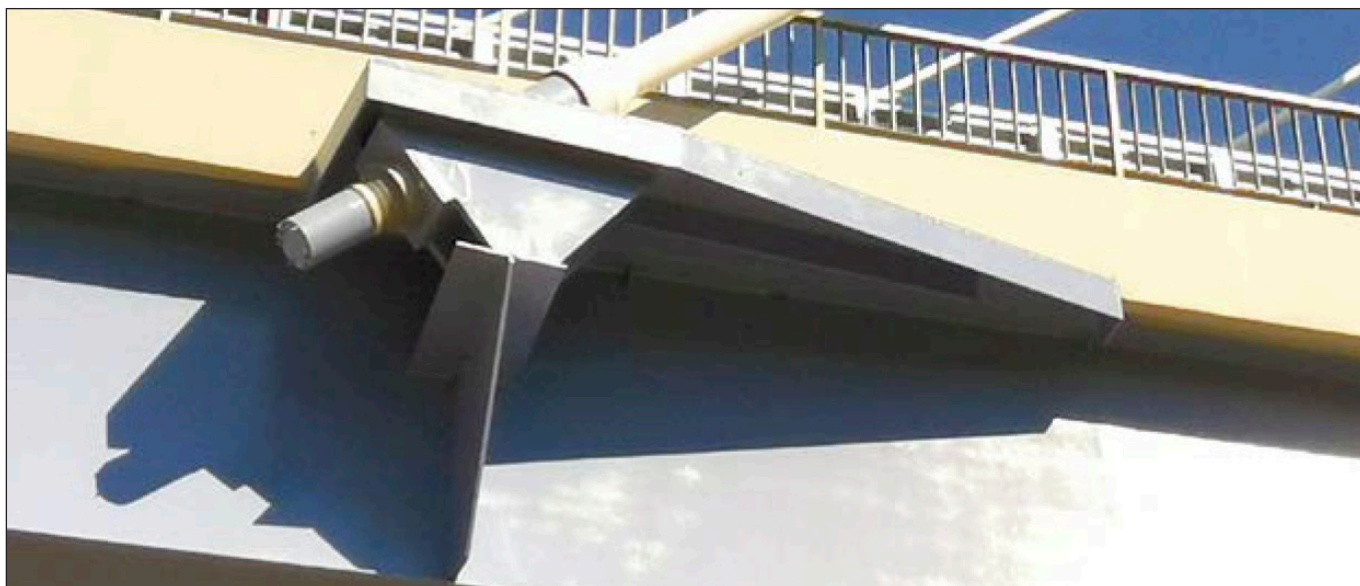
Fig. 3: Cable anchoring cantilever of the stiffening girder
