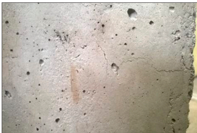
Fig. 4: Crack lines formed on 15% recycled concrete after tempering for 2 hours at 400 °C (Salau et al., 2015)
