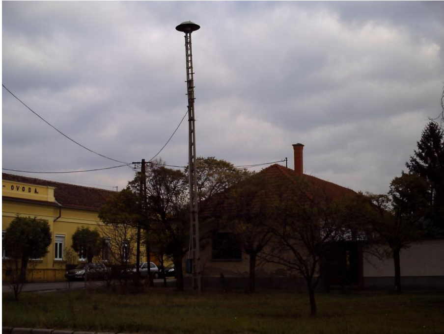
Installed residential alert terminus, disaster management powered siren Source: Szentés Civil Protection Branch
