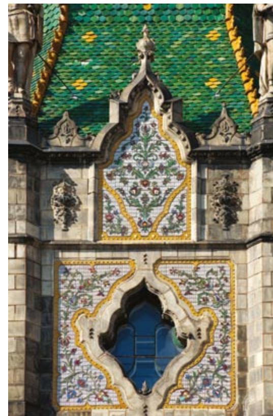
Museum of Applied Arts, Budapest Floral patterned ceramic ornamentation on the facade
