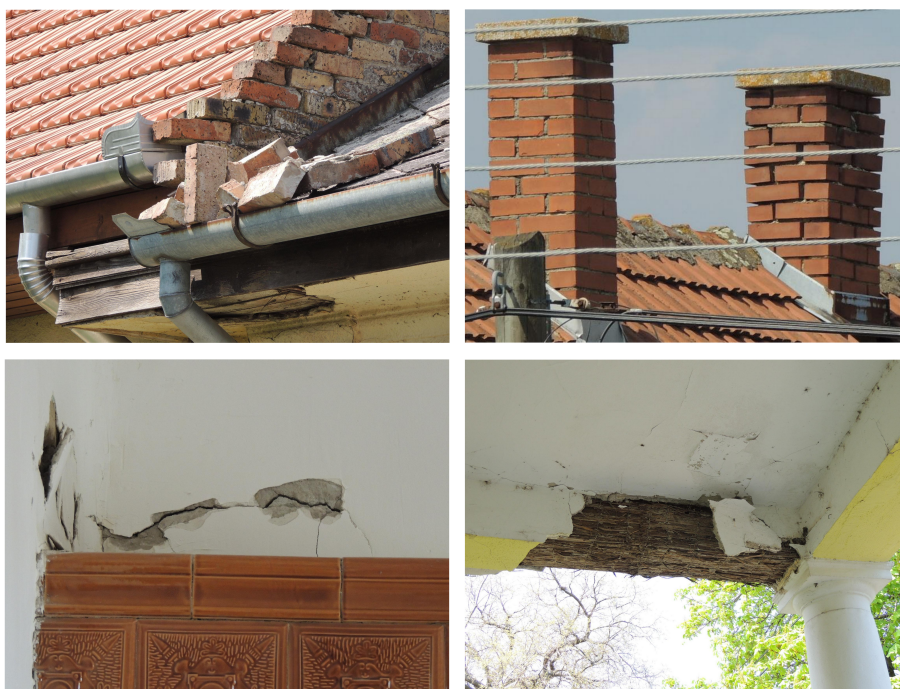
Fig. 5 Characteristic building damages in Tenk. (Photos: Erzsébet Gyóri)
