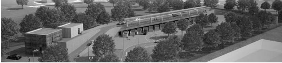
Picture 2. Lamusownia – modern waste facility. 15
