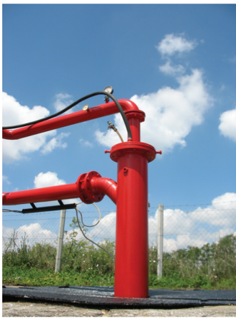
Figure 2. Thermal well with diving-pump excavation
