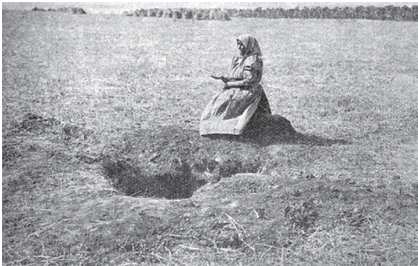
Fig. 6 The place of dug up sand volcano generated during 1911 Kecskemét earthquake (photo from MTA CSFK GGI Archive)
